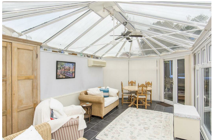
UPVC double-glazed construction with double-glazed roof. Air conditioning unit. Tiled flooring. Radiator.
