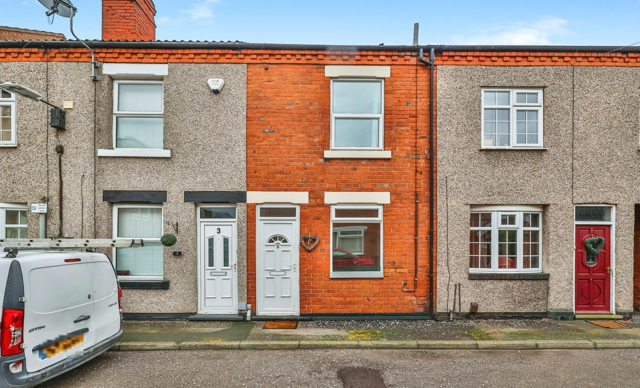
Titchfield Terrace Hucknall Nottingham
