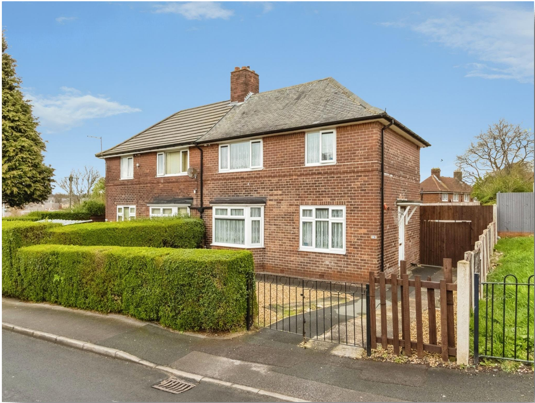
Mardale Crescent, Leeds LS14 6DP
