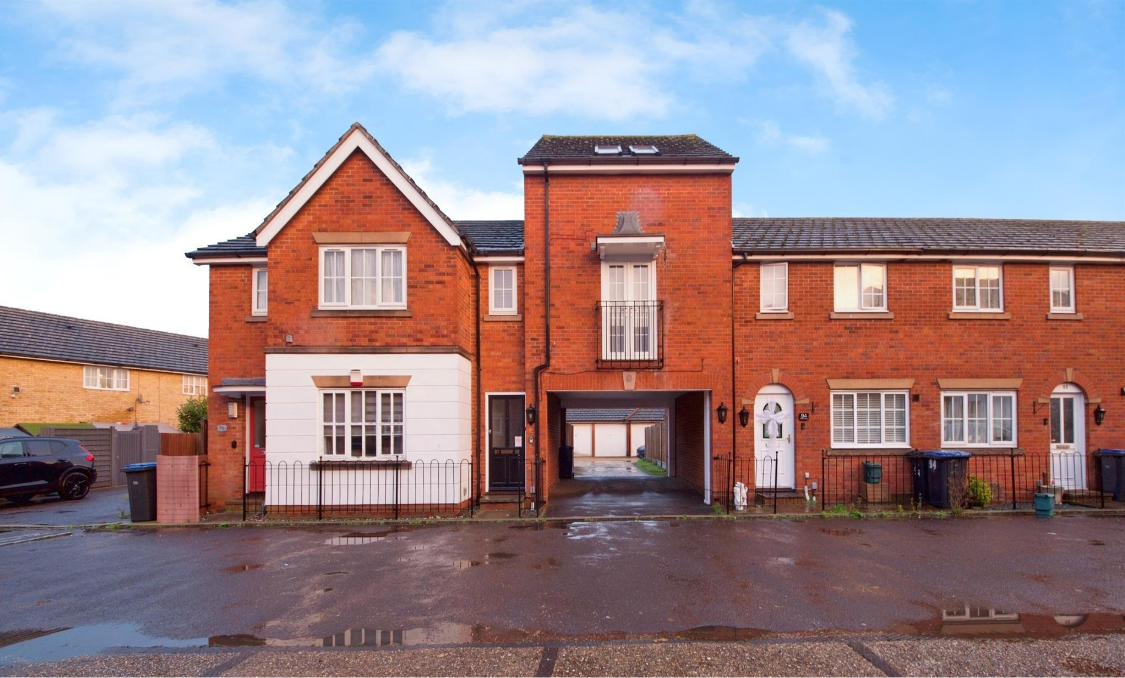
Hadley Grange, HARLOW CM17 9PH
