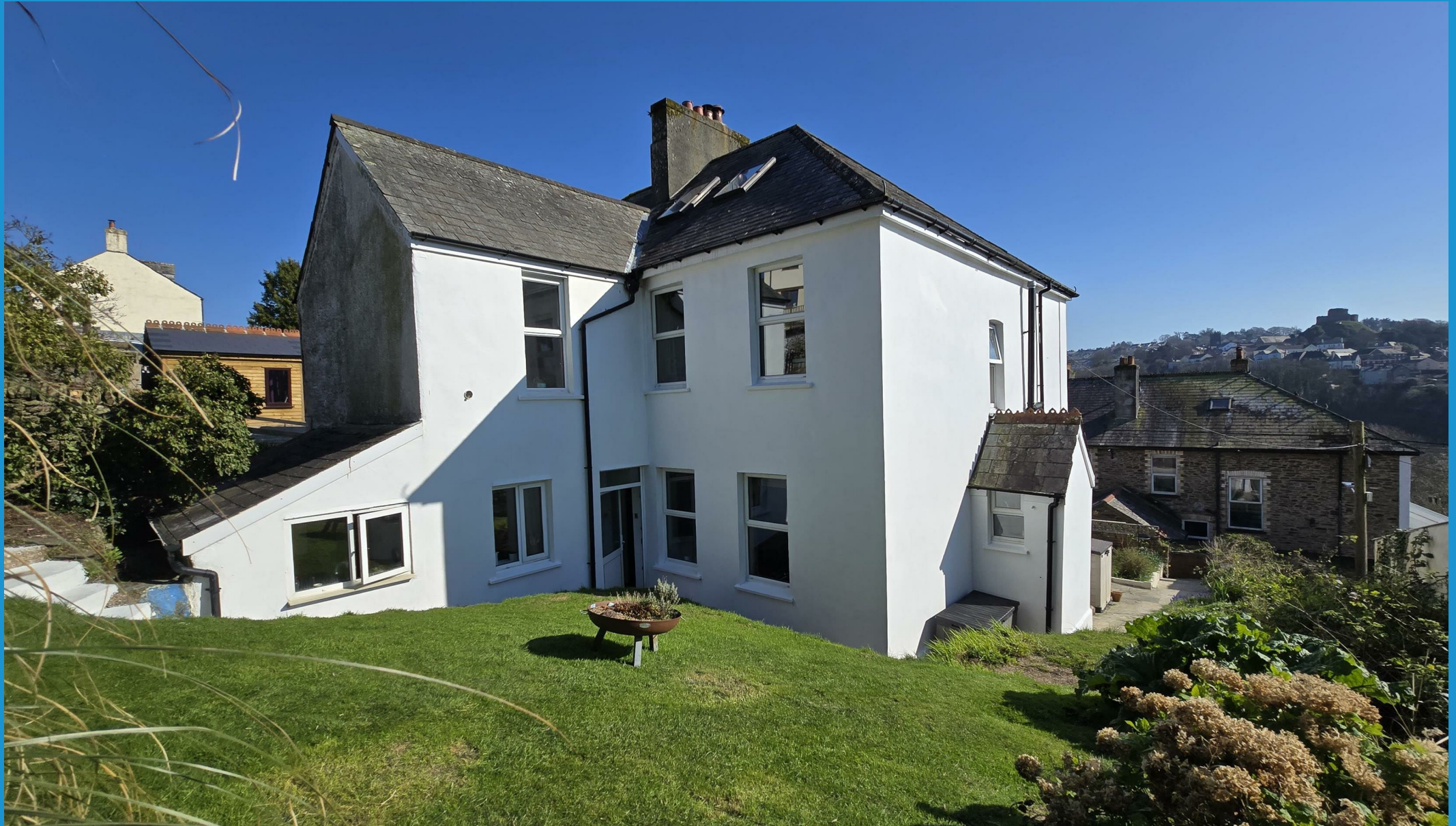
Dutson Road Launceston | Cornwall
