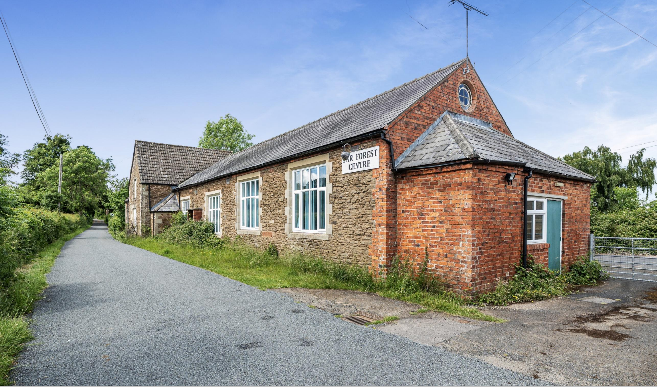
Former Far Forest Community Centre, Church Lane, Far Forest, Kidderminster, DY14 9TP
