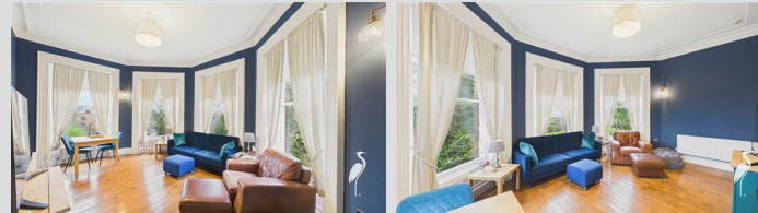
4x single glazed windows and 3x double radiators.
