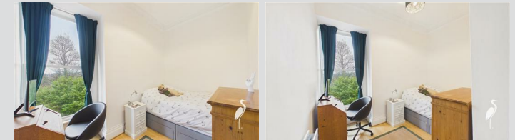
Single glazed window and double radiator.
