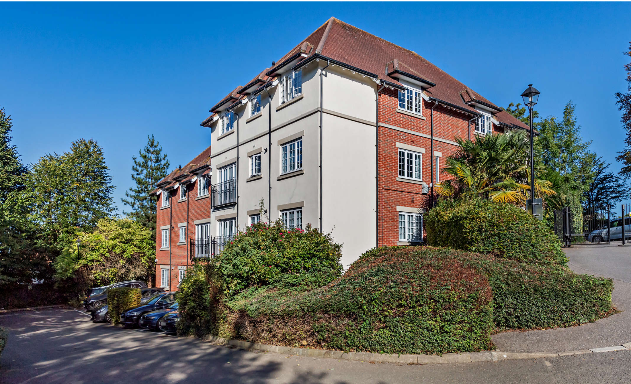
A two bedroom apartment in a gated development Sycamore Lodge, Cottage Close, HA2 0HA
