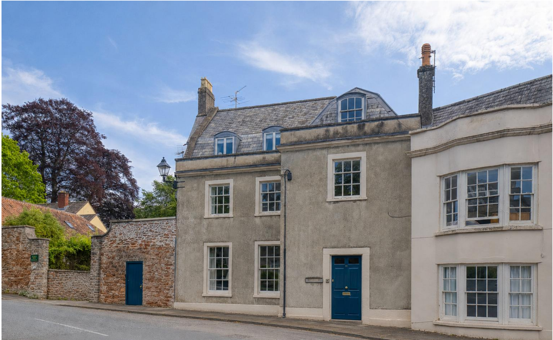
The Hollies, Wells
