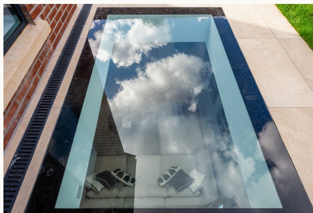
Glass roof-light set into the patio · 花园露台上嵌玻璃天窗
