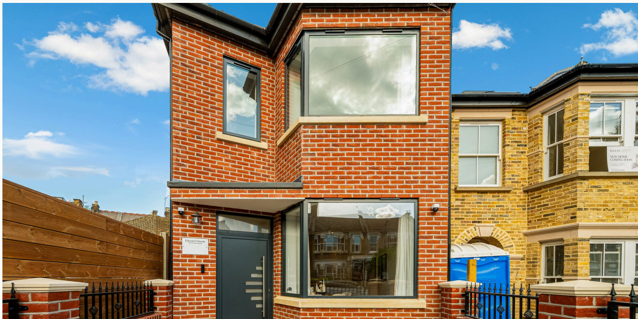
Eduard House, Kings Road — front elevation behind a gated, iron-railed entrance · 正立面，铁艺围栏与门禁入口
