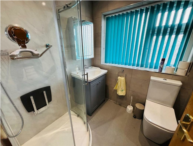
Double glazed window, glazed shower cubicle with a shower above, low flush WC, wash basin set into a vanity unit, central heating radiator / towel warmer
