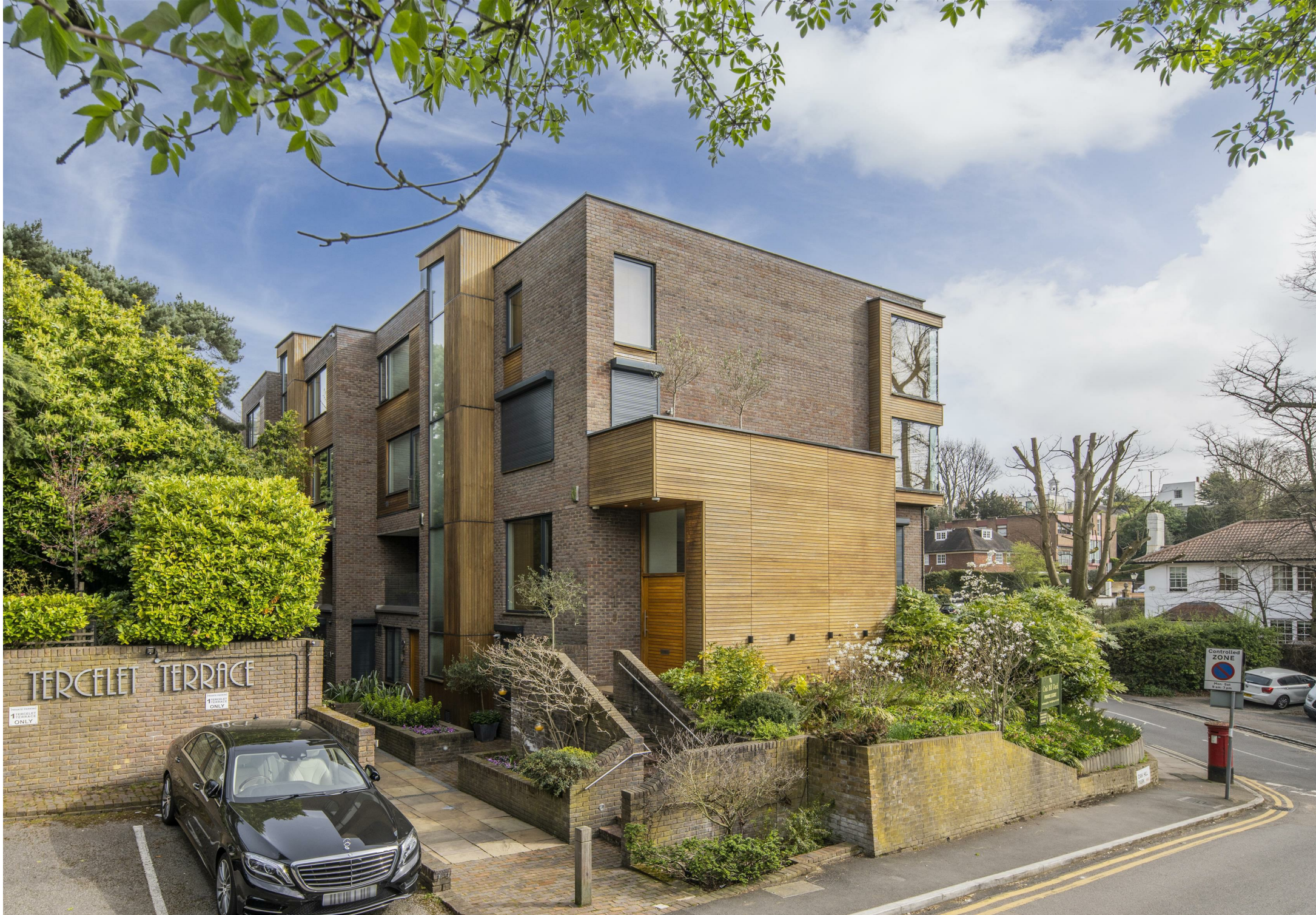
The front exterior photograph is provided to illustrate the general exterior of the houses in the terrace and parking area.
