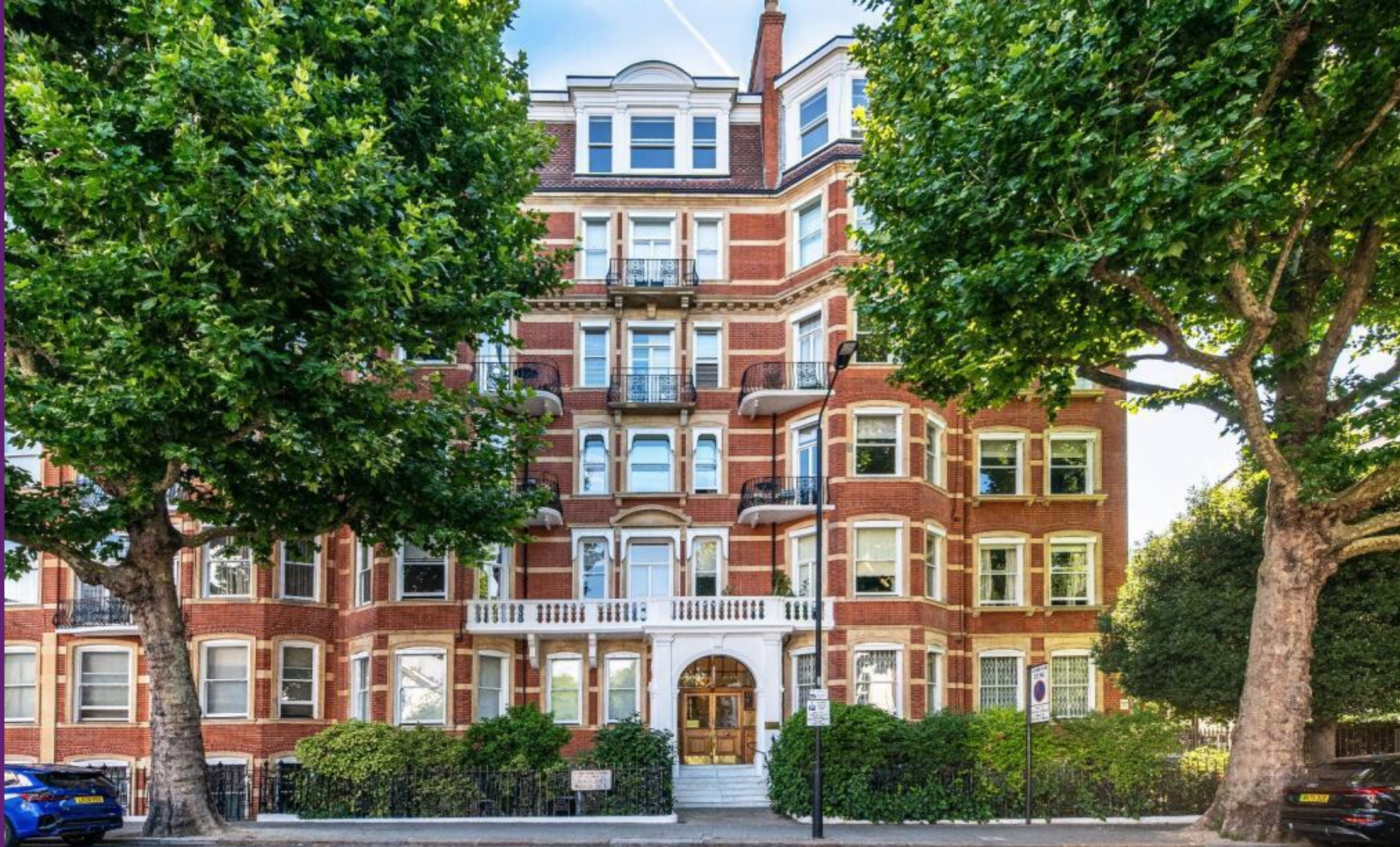
Sutherland House Marloes Road, W8
