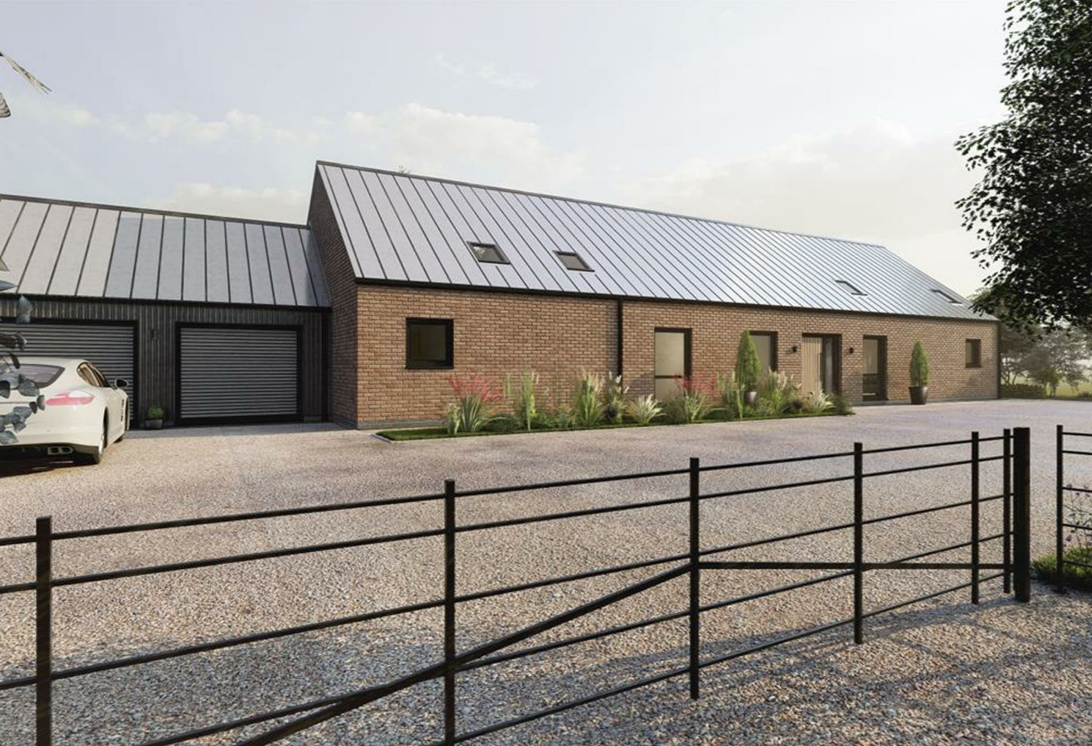
BARN 3 BEECHES FARM, BRADBOURNE FRONT ASPECT
