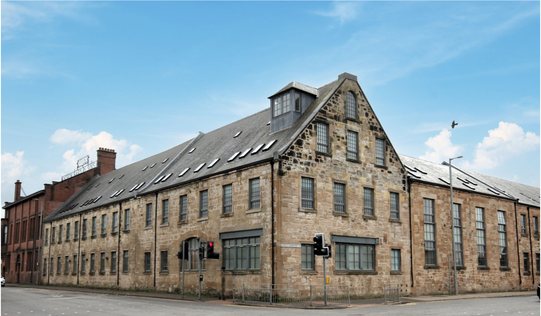
Apartment 15, Barclay House, West Langlands Street, Kilmarnock, KA1 2PR Offers Over £85,000
