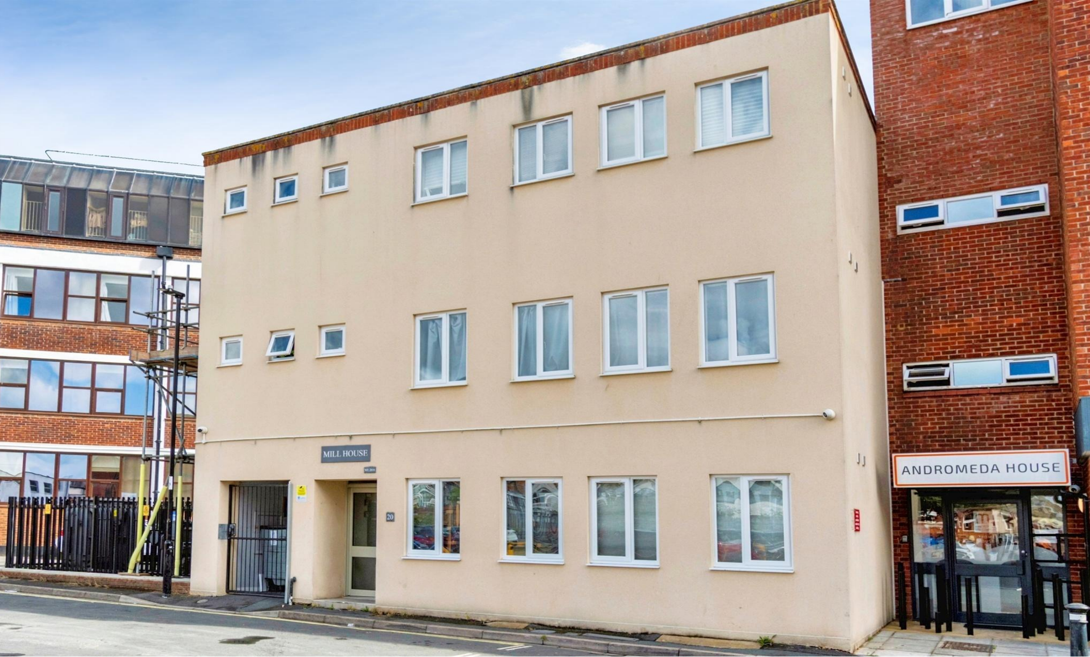
Mill House, Southampton Street, Southampton SO15 2ED
