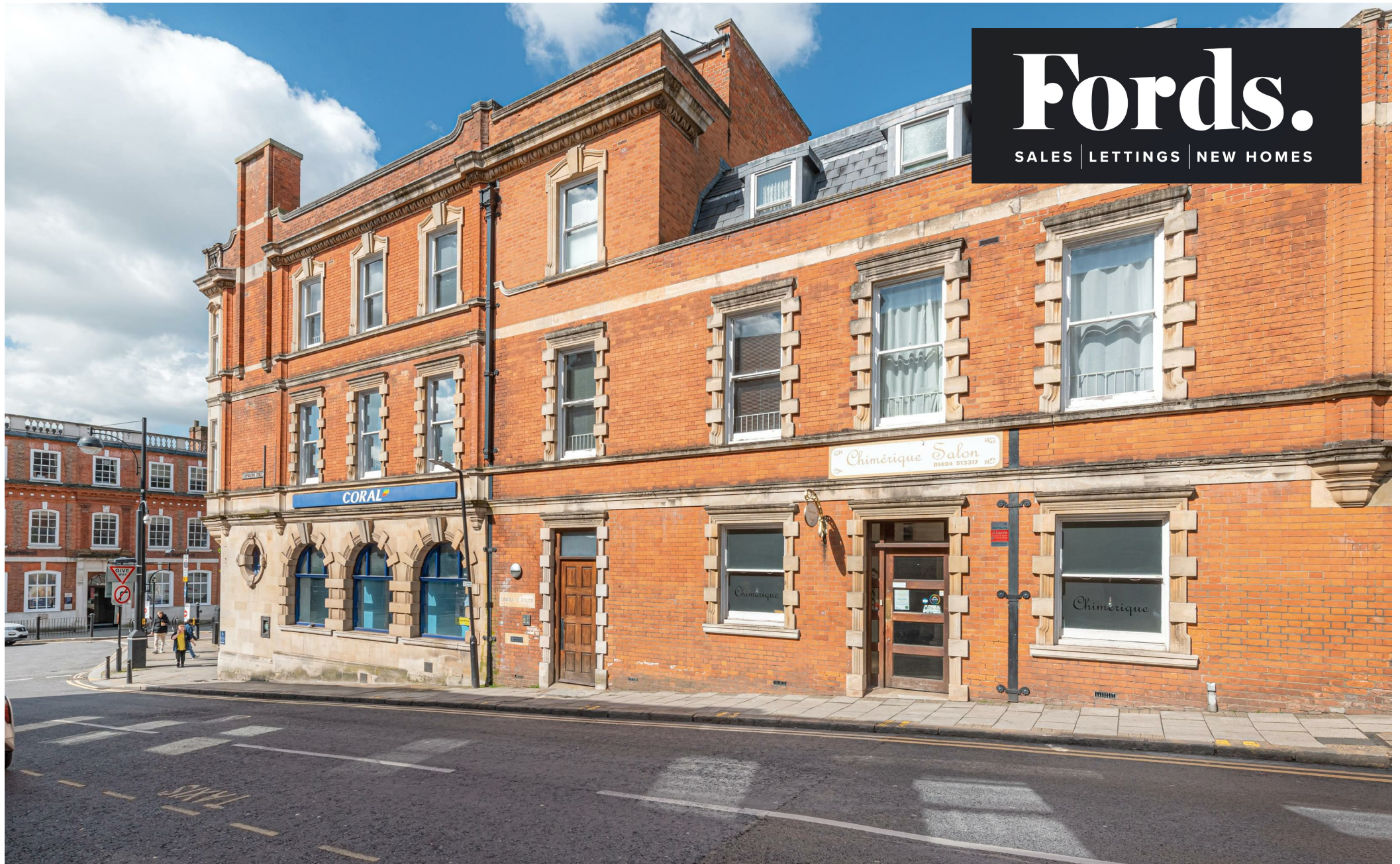
Old Bank House, 1 Corporation Street, High Wycombe, Buckinghamshire, HP13 6TQ
