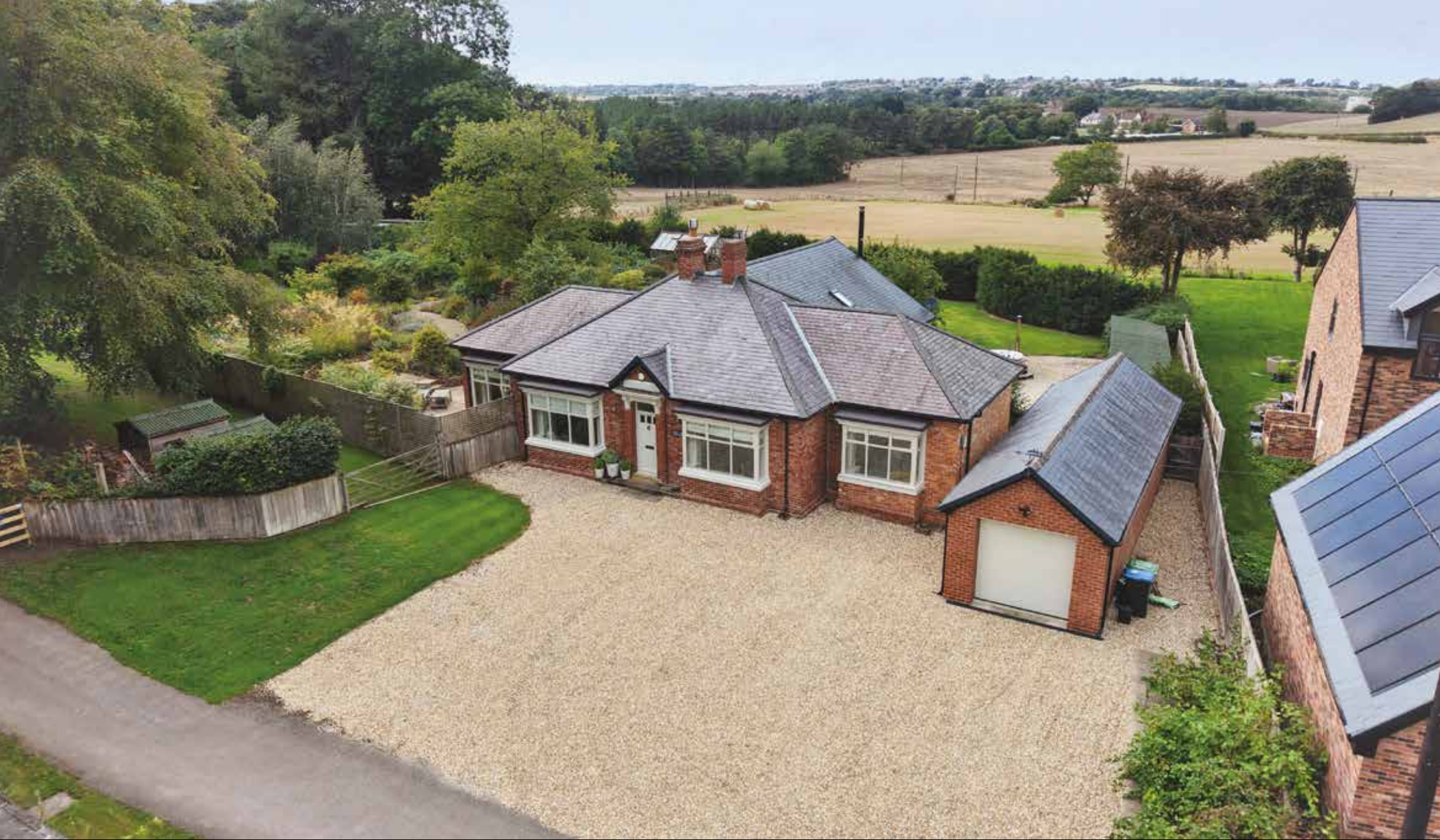
Nable Hill Cottage Mainsforth | Ferryhill | County Durham | DL17 9AA
