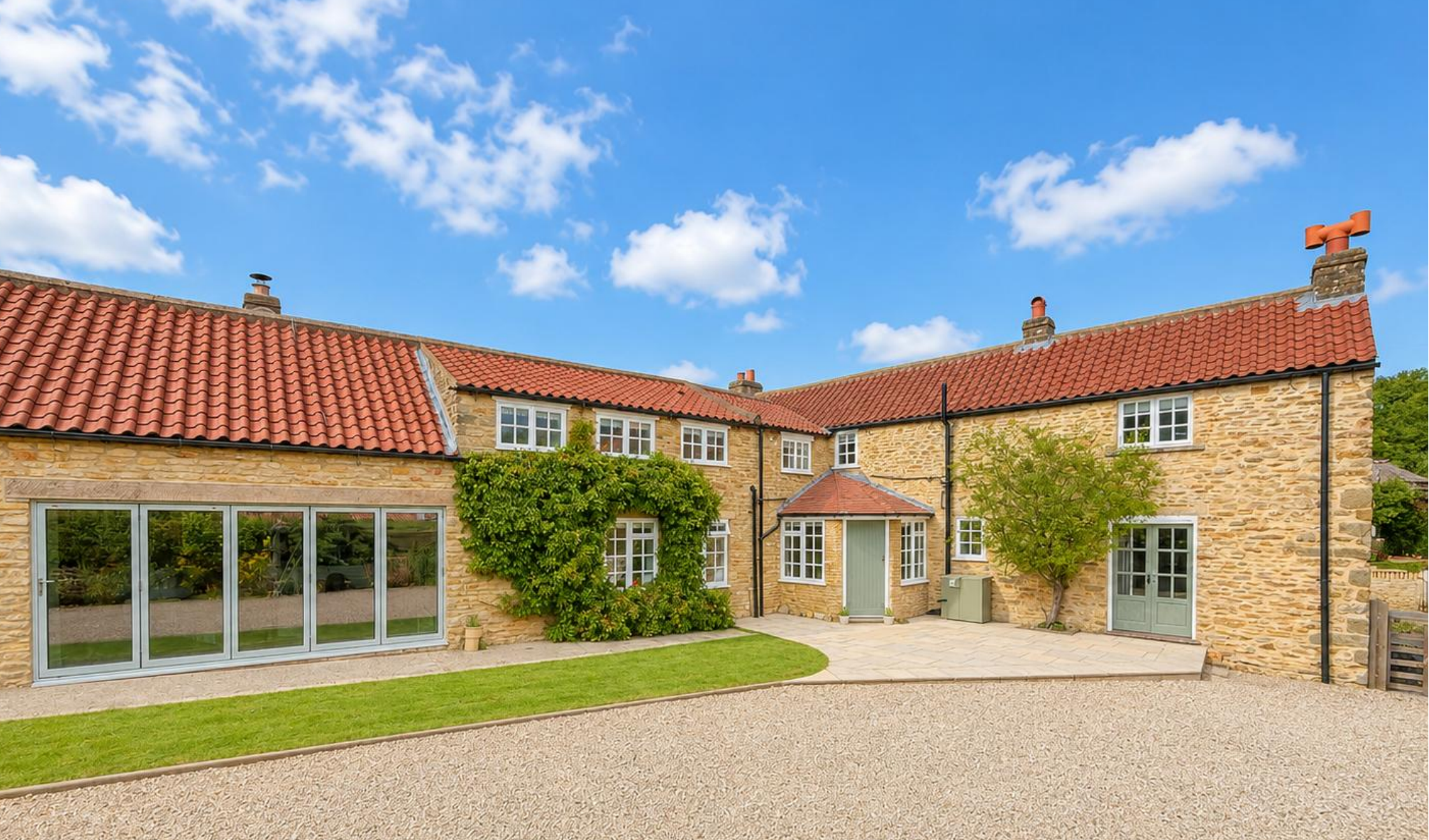
HOLLY COTTAGE SAWDON, NORTH YORKSHIRE
