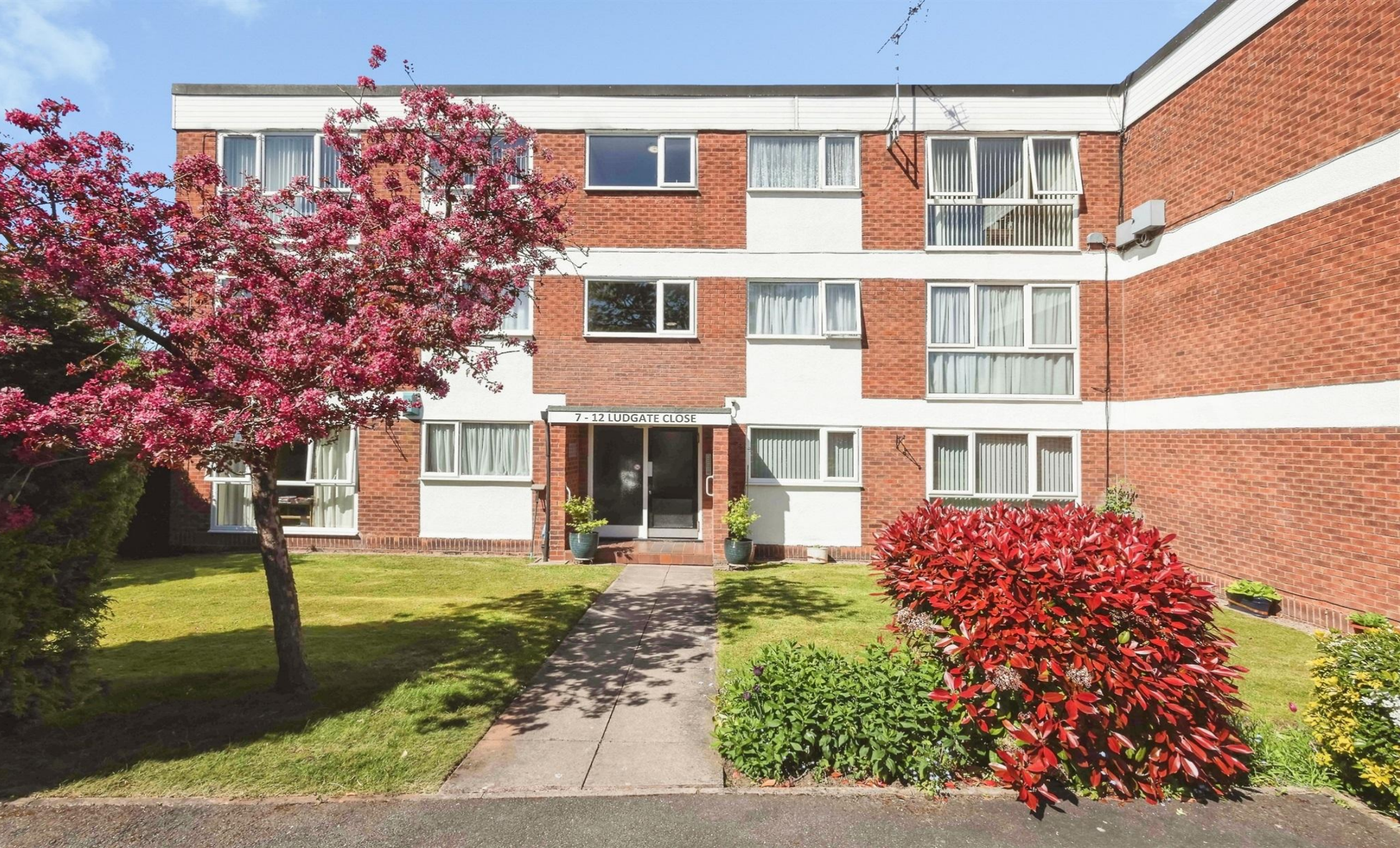
Ludgate Close, Water Orton, BIRMINGHAM
