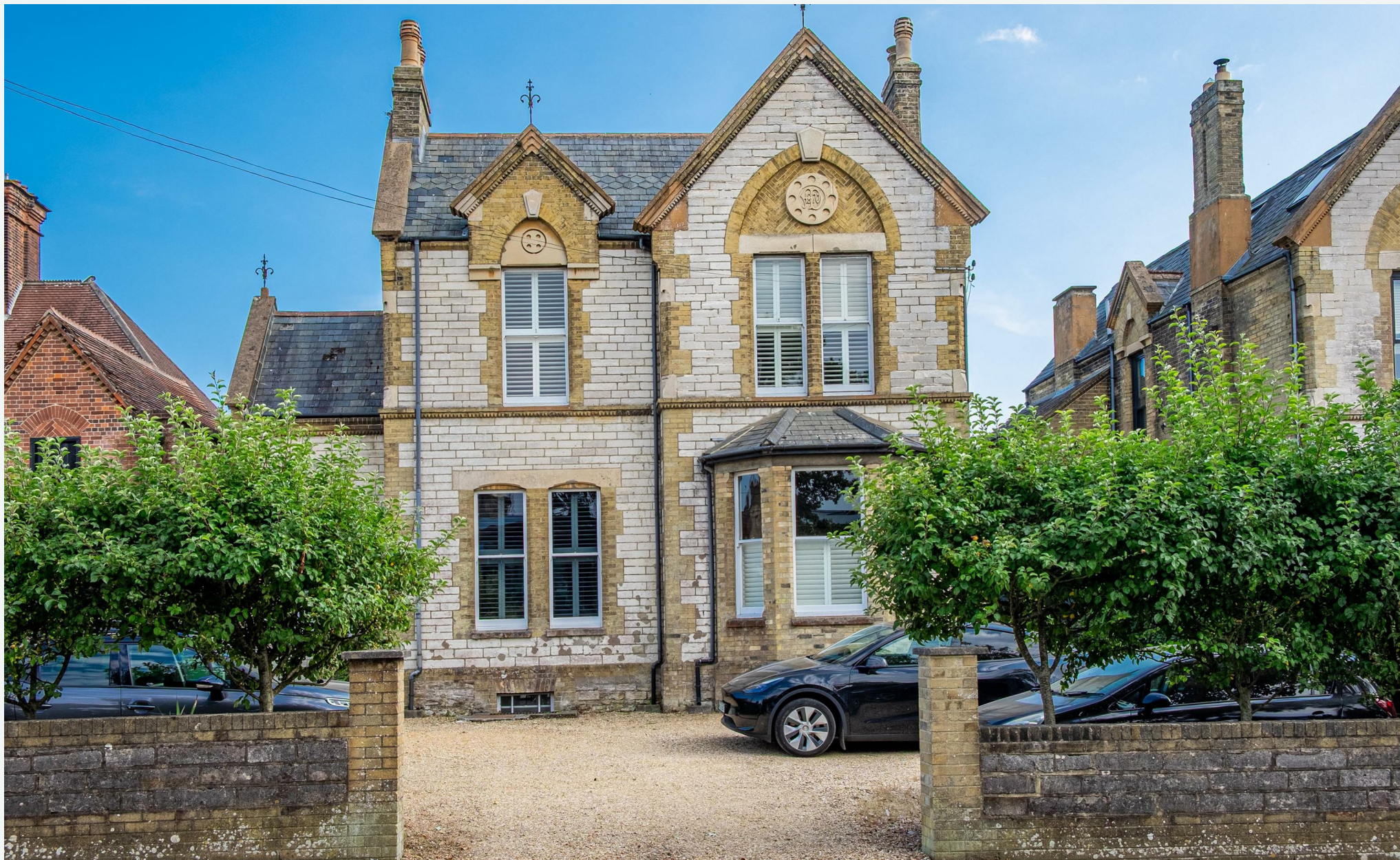
Hafod, Queens Road, Ryde, Isle Of Wight, PO33 3BG
