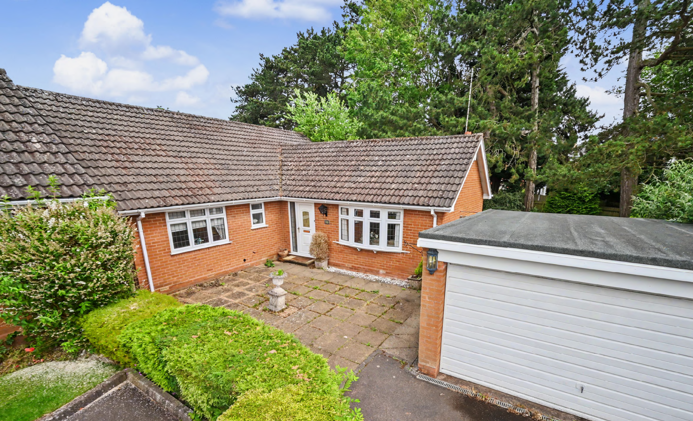
28 Saxon Court, Tettenhall
