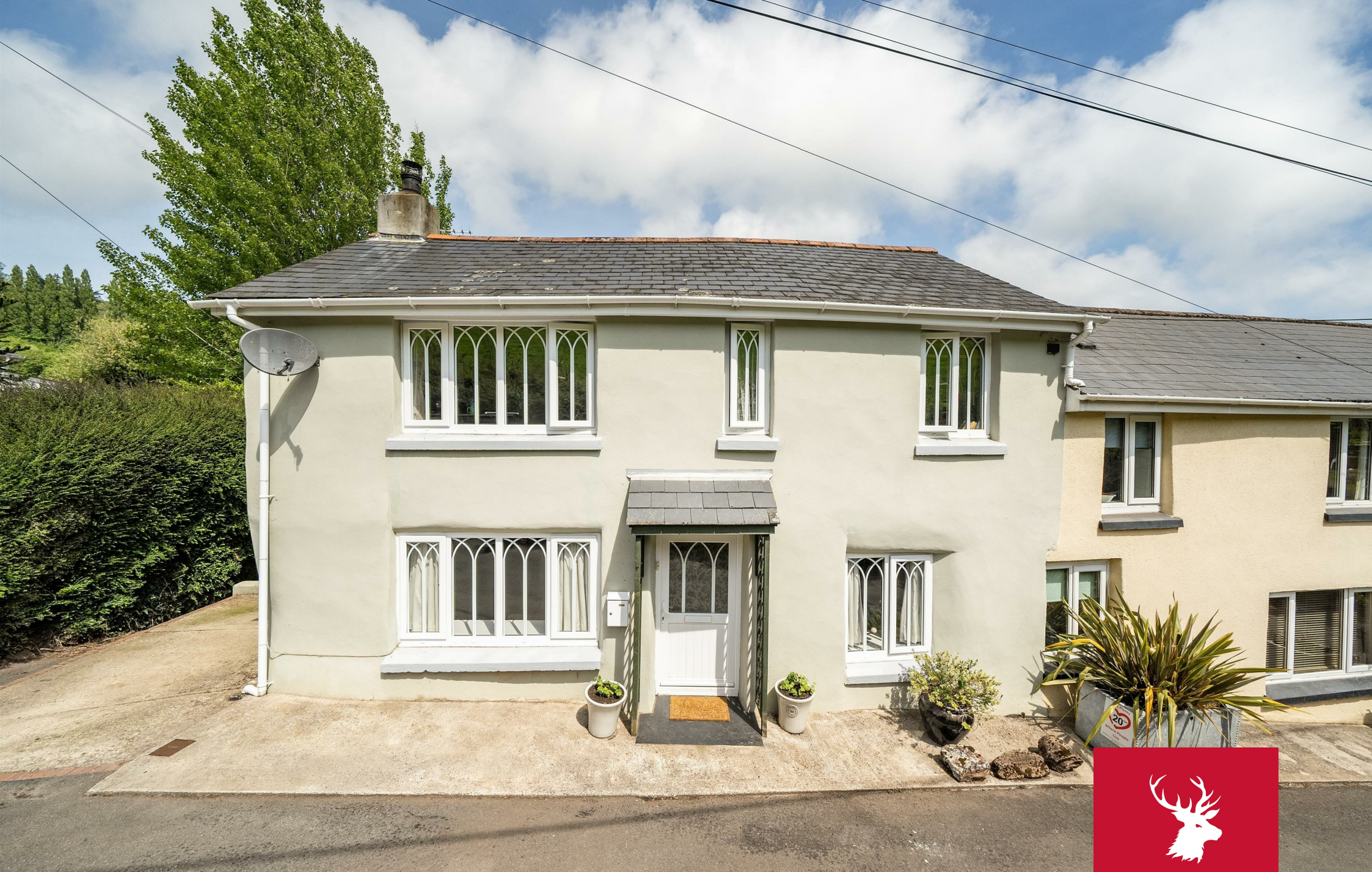
1 Coombe Cottages, Coombe Way
