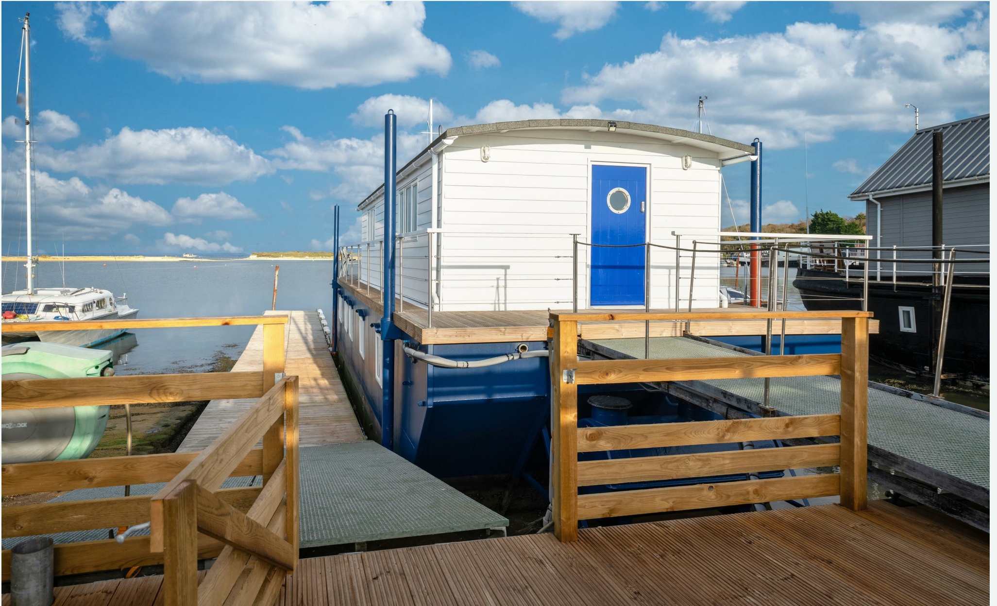
Houseboat Oystercatcher, Embankment Road, Bembridge, PO35 5NS
