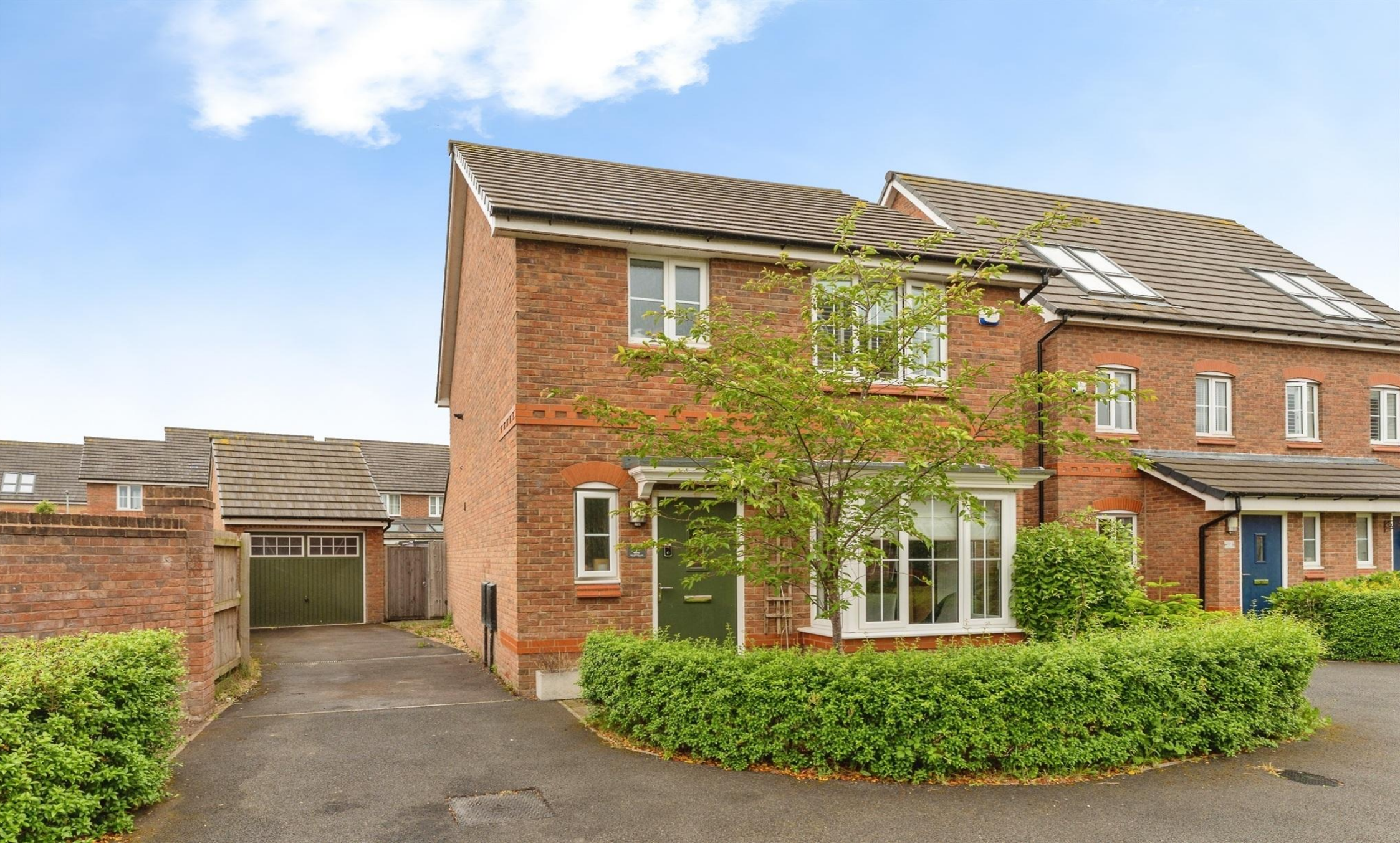
Oxford Court, Sealand Deeside CH5 2FR
