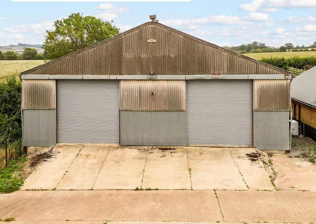
Existing Barn: Front Elevation
