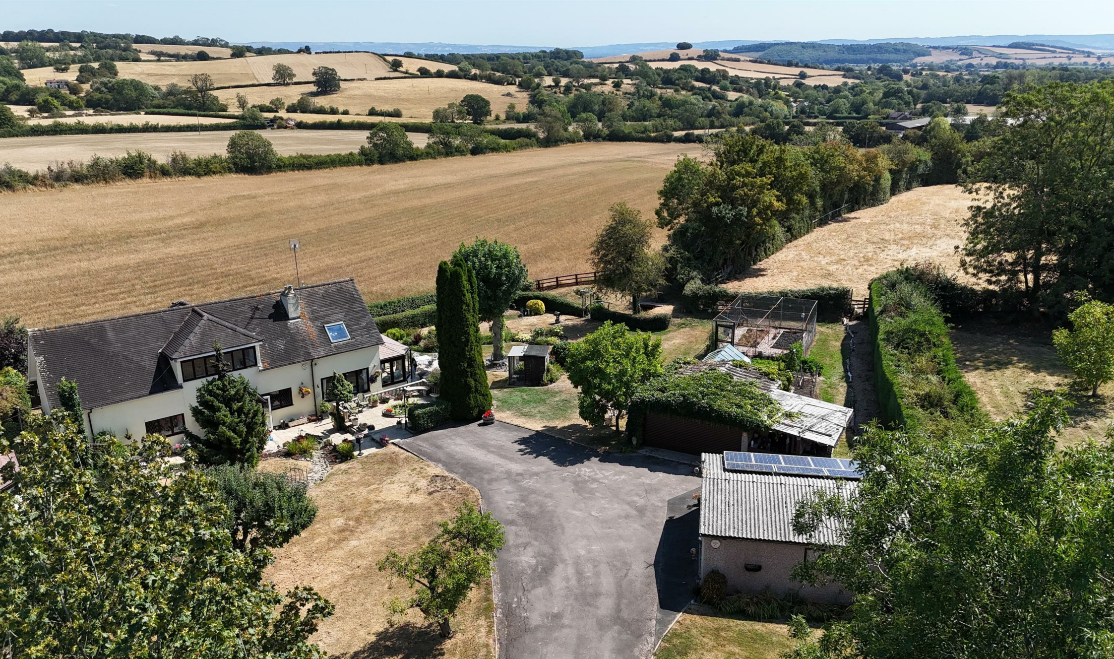
Ivy Cottage Upper Hasfield, Hasfield GL19 4LL
