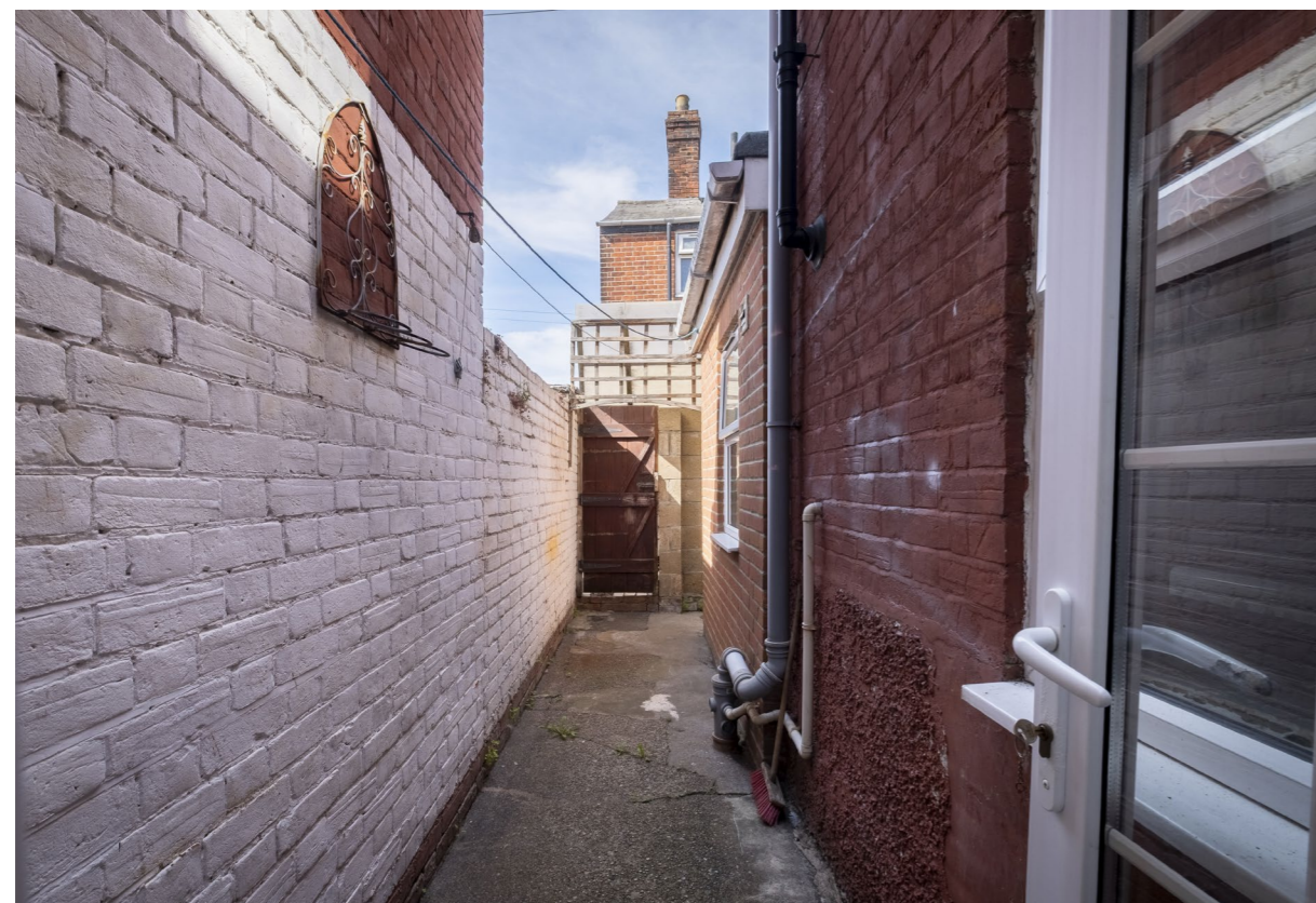
West facing rear yard
