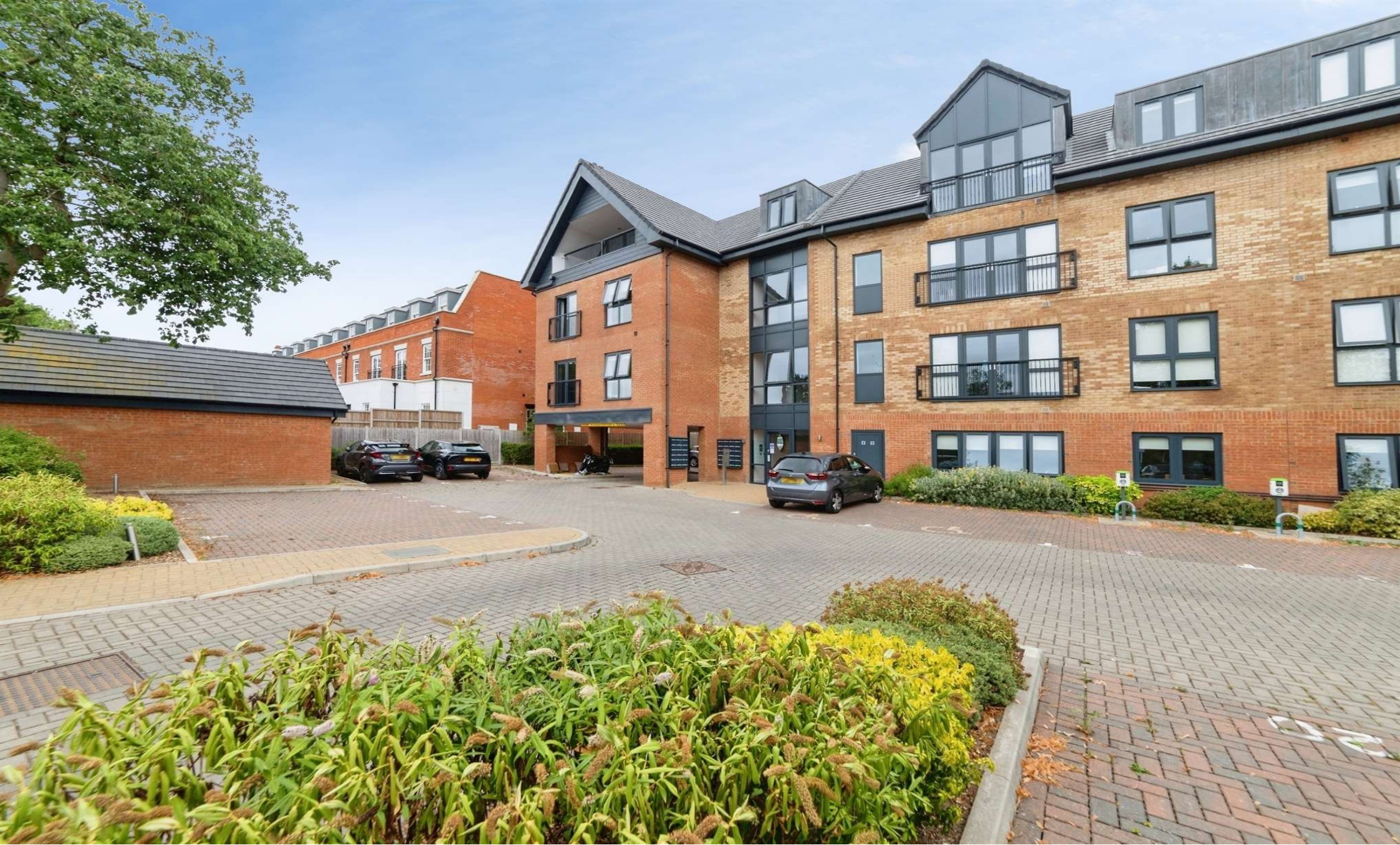
De Havilland House, North Road, Stevenage, SG1 4FU
