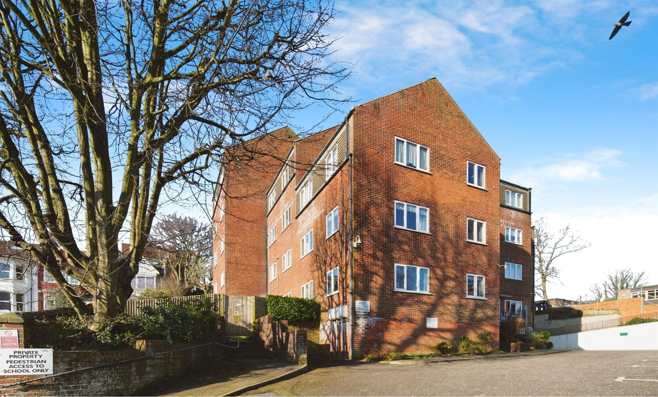
Elm Court Dyke Road, Brighton BN1 5AX
