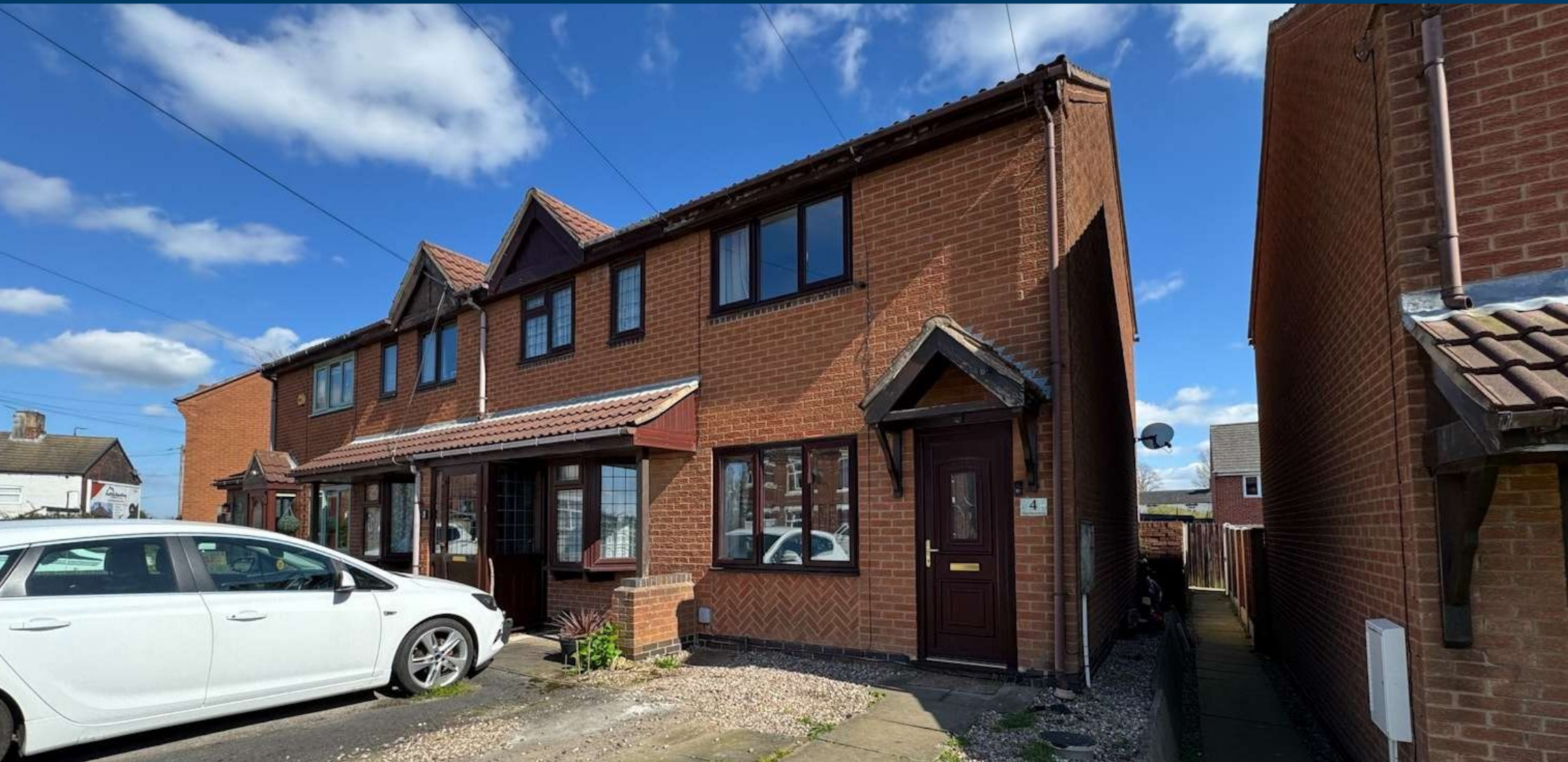
Thorn Street Mews Thorn Street, Woodville, Swadlincote, Derbyshire
