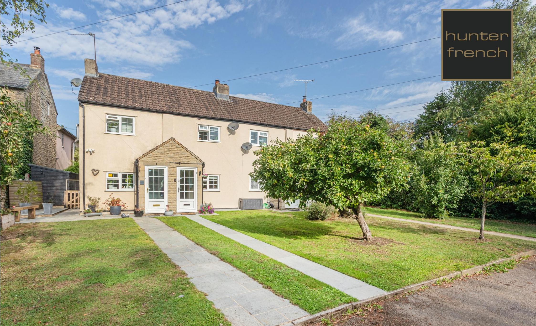
2 Home Farm Cottages, Burton Hill, Malmesbury, Wiltshire, SN16 0EW
