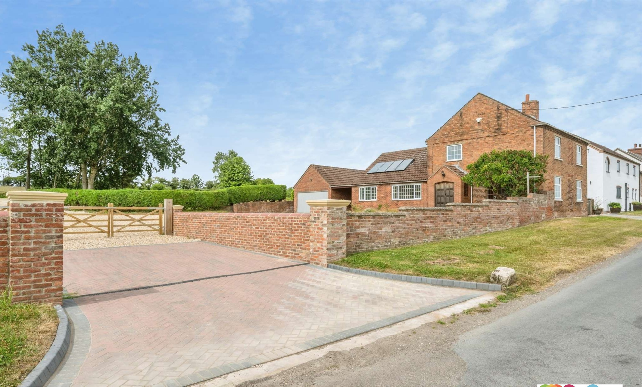
Harwell House, Middle Bridge Road, Gringley-On-The-Hill Doncaster DN10 4SD
