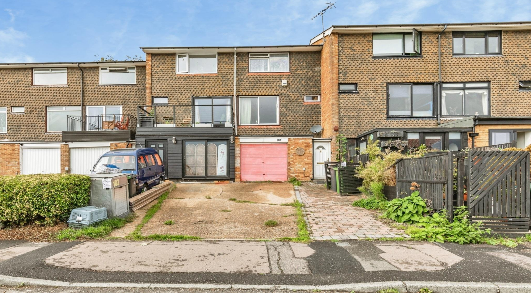
Bembrook Road, Hastings TN34 3PB
