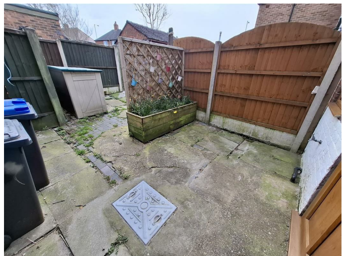
To the rear of the property is a back yard with shared access together with a small outbuilding (former WC).
