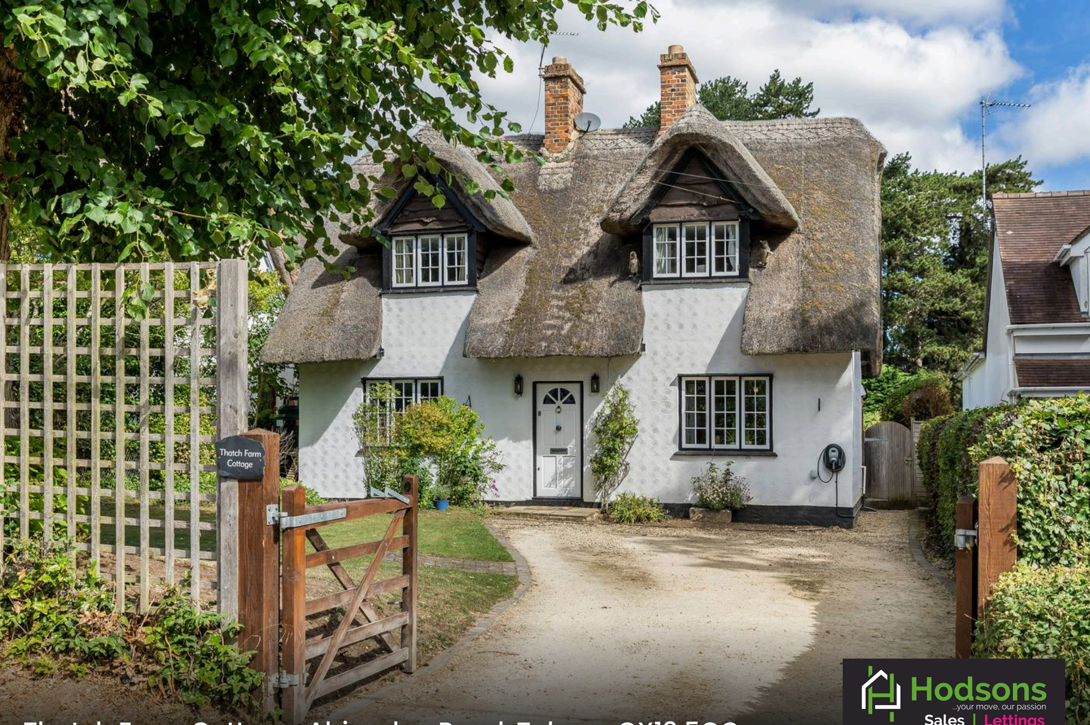
Thatch Farm Cottage, Abingdon Road, Tubney OX13 5QQ
