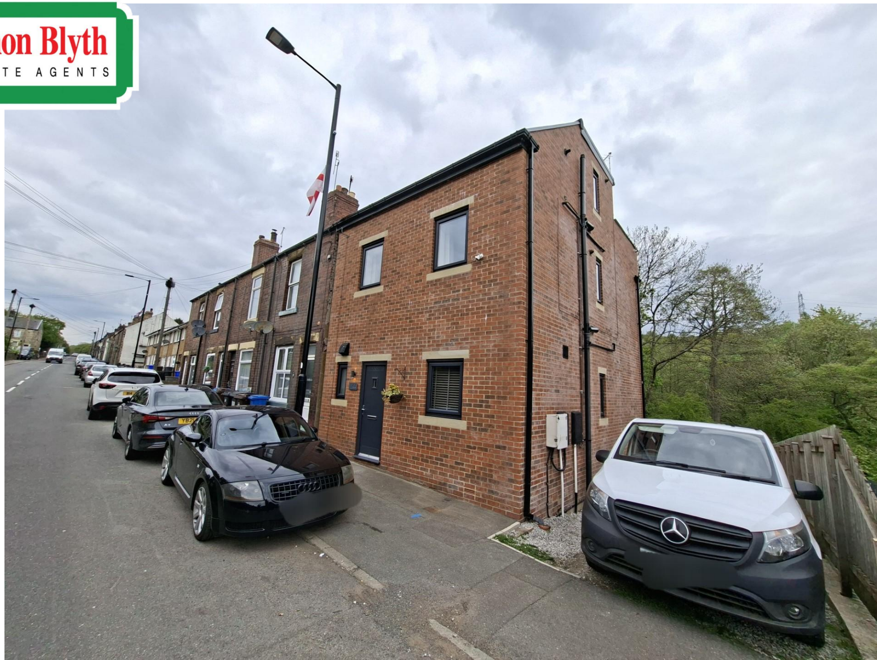
MANCHESTER ROAD, DEEPCAR, S36 2RE
