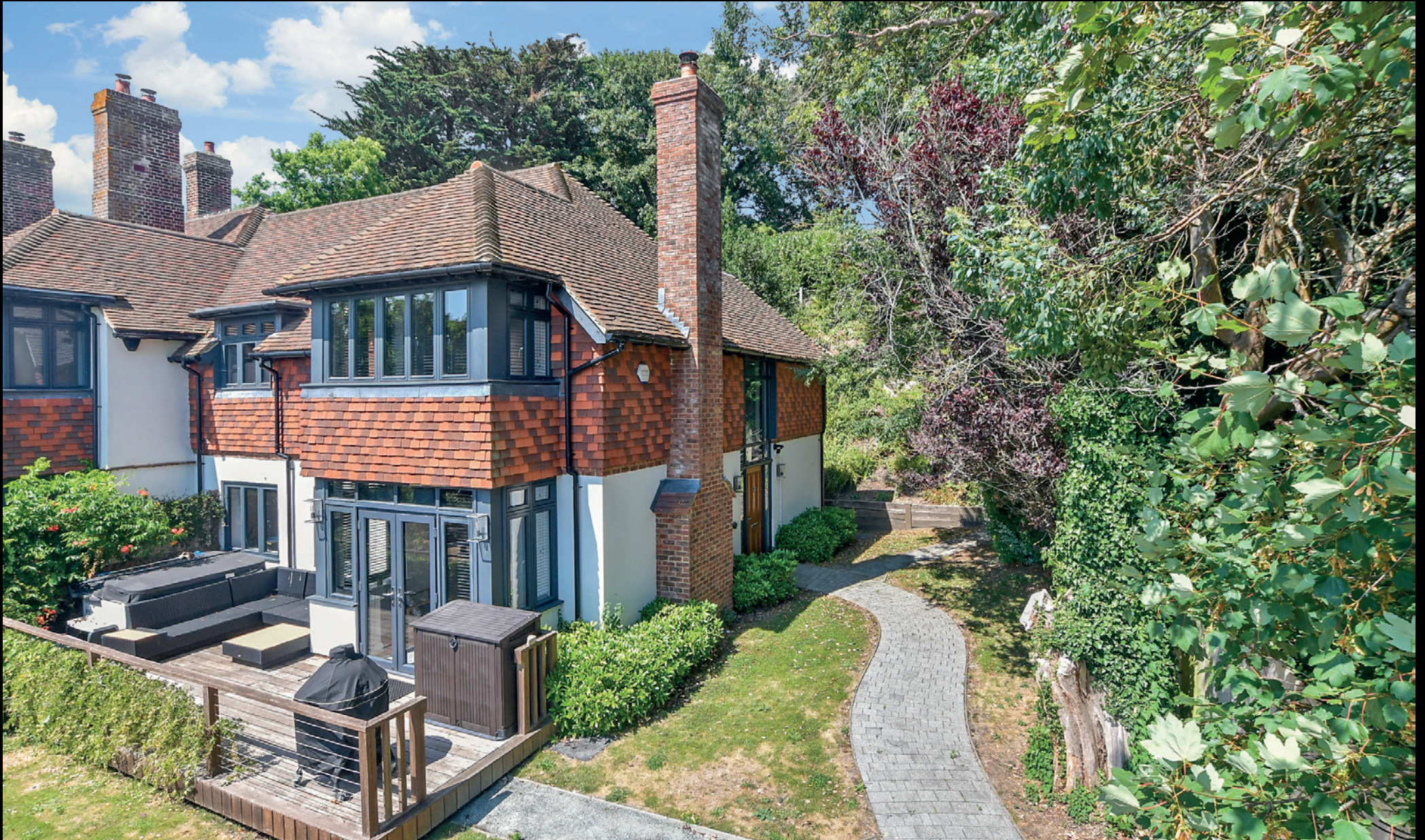
3 Haverfield House Cannongate Road | Hythe | Kent | CT21 5PX
