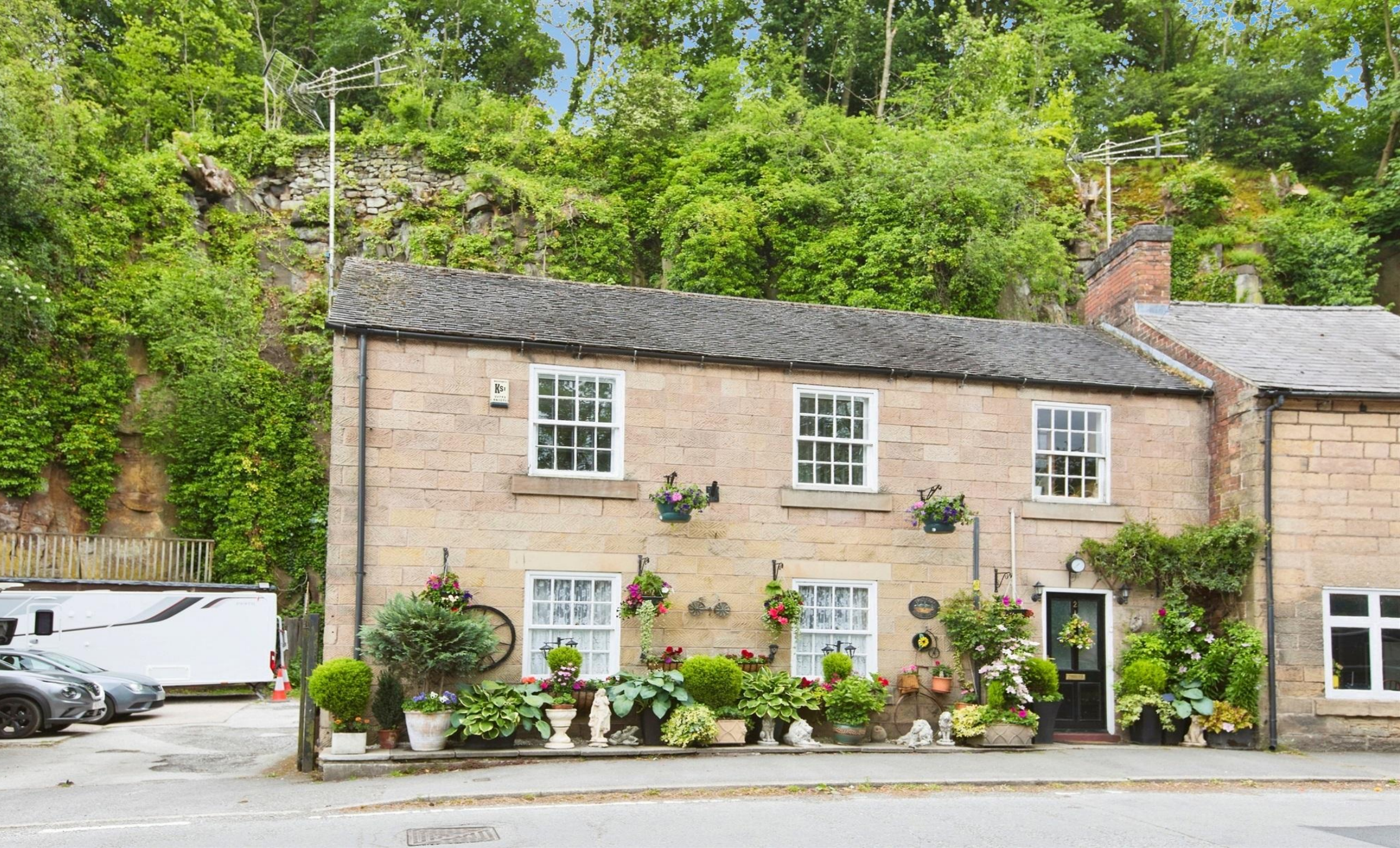
The Old Bike Shop 1a The Bridge Milford BELPER
