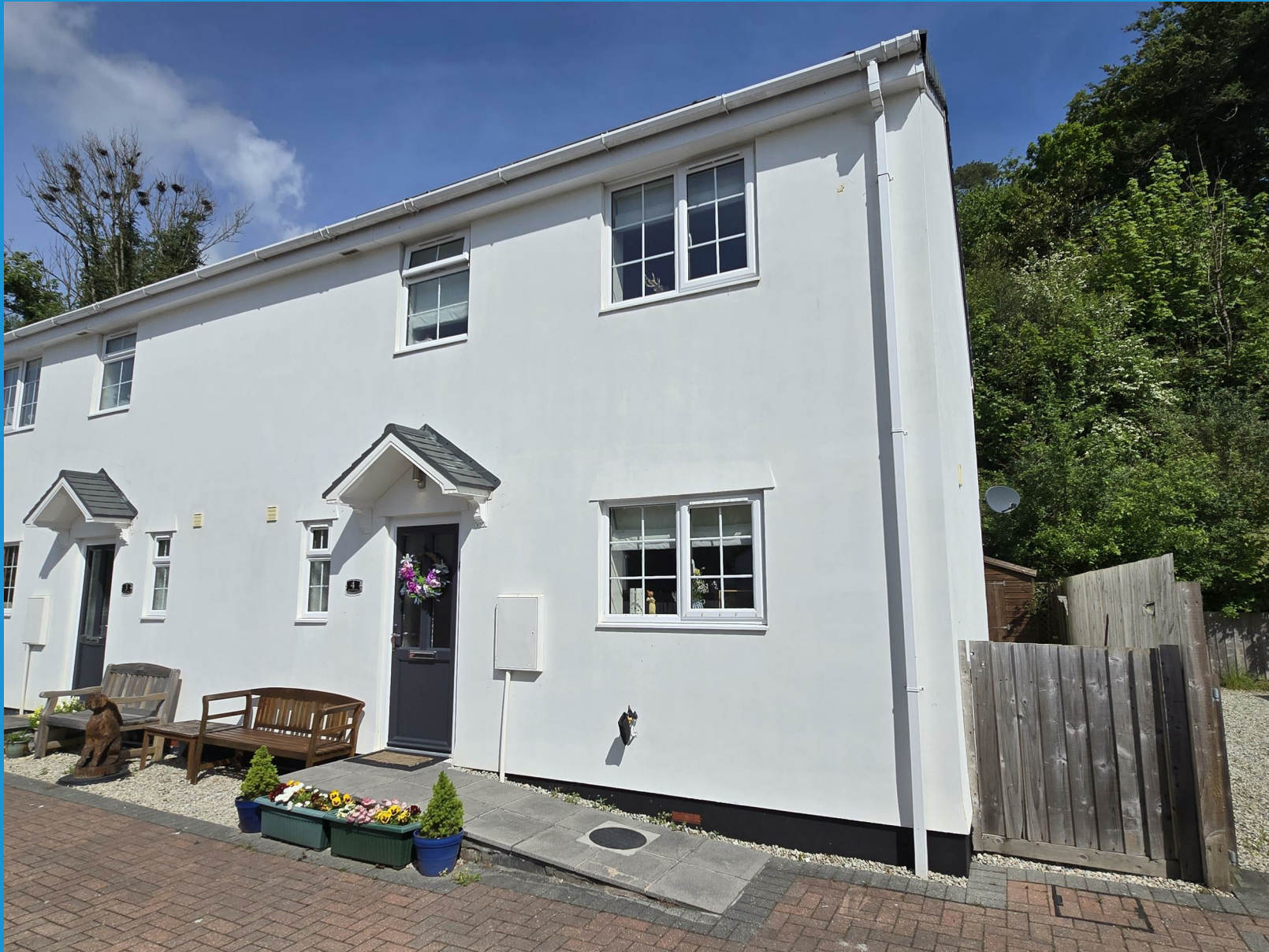
4, The Lime Kilns Lifton | Devon
