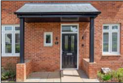
Sloping Porch and Front Door
