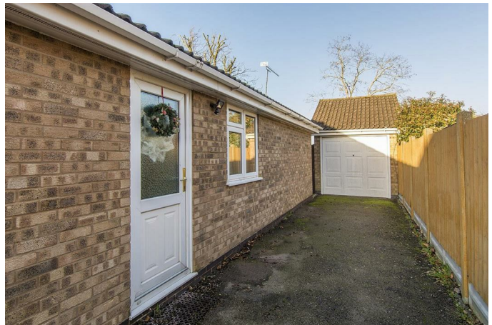
Up and over vehicle access door. Power and light connected.
