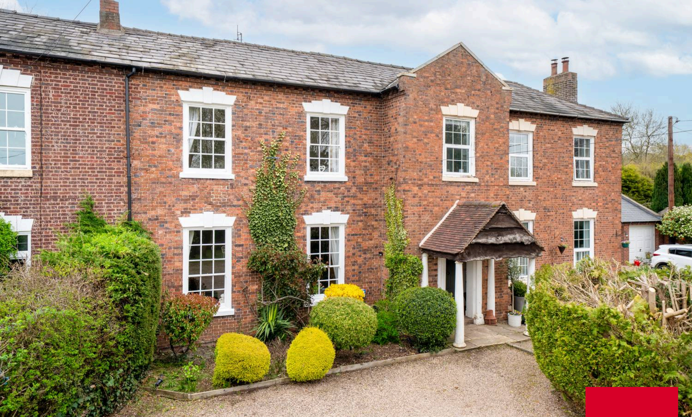
1 Beechcote House, Mill Lane, Wolverley, DY11 5TR
