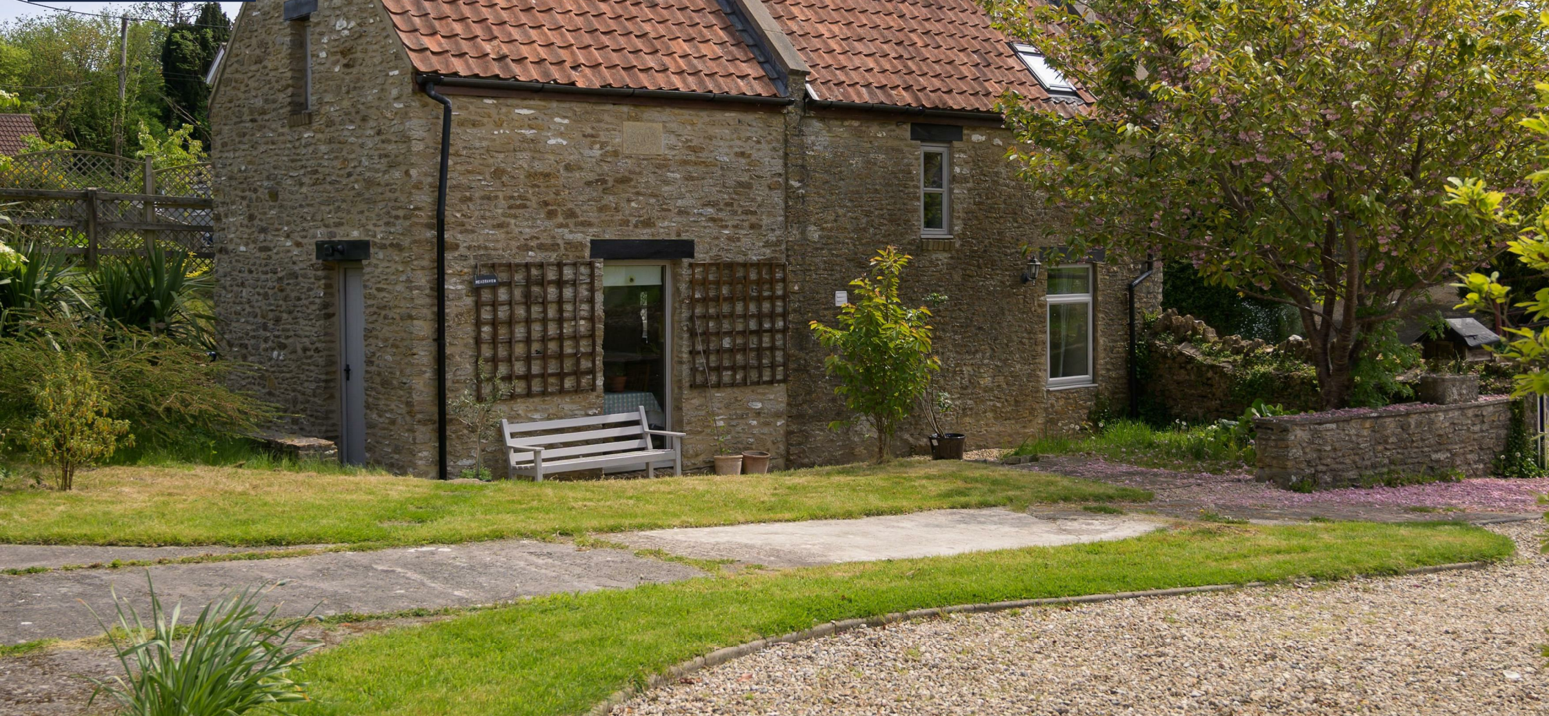
The Gardeners Lodge, Riverside Cottage, Wanstrow
