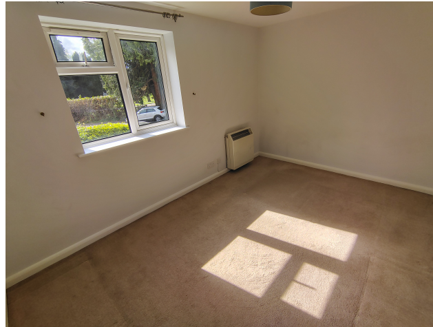
BEDROOM ONE electric heater
