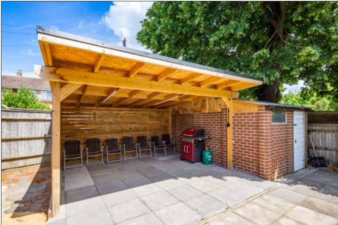
Rear Covered BBQ/Entertaining Area
