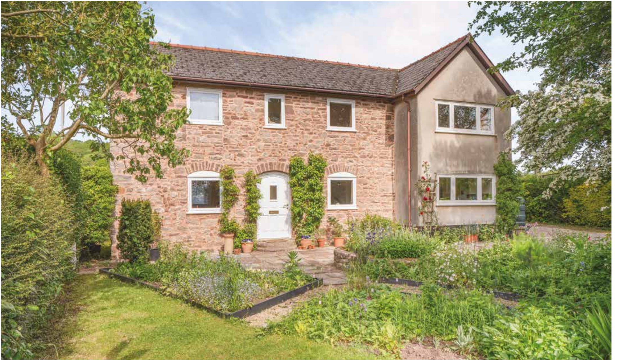
Corner Cottage Woodside | Woolaston | Gloucestershire | GL15 6PA
