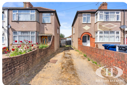
DRIVEWAY & SIDE ACCESS
