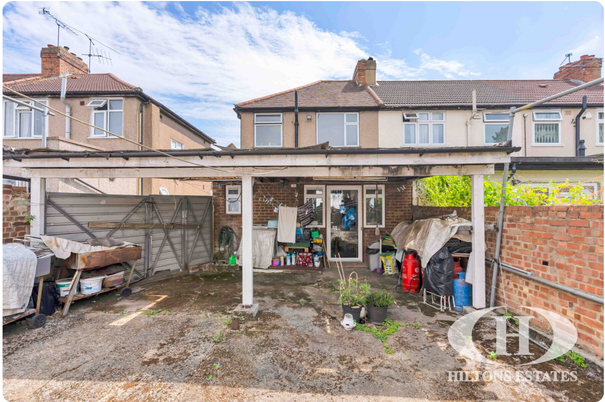
REAR OF HOUSE
