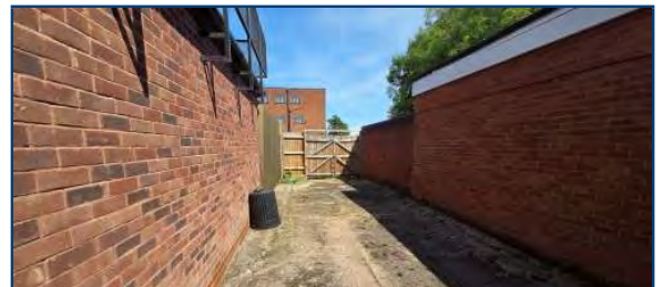
Gated Yard providing Off Road Parking
