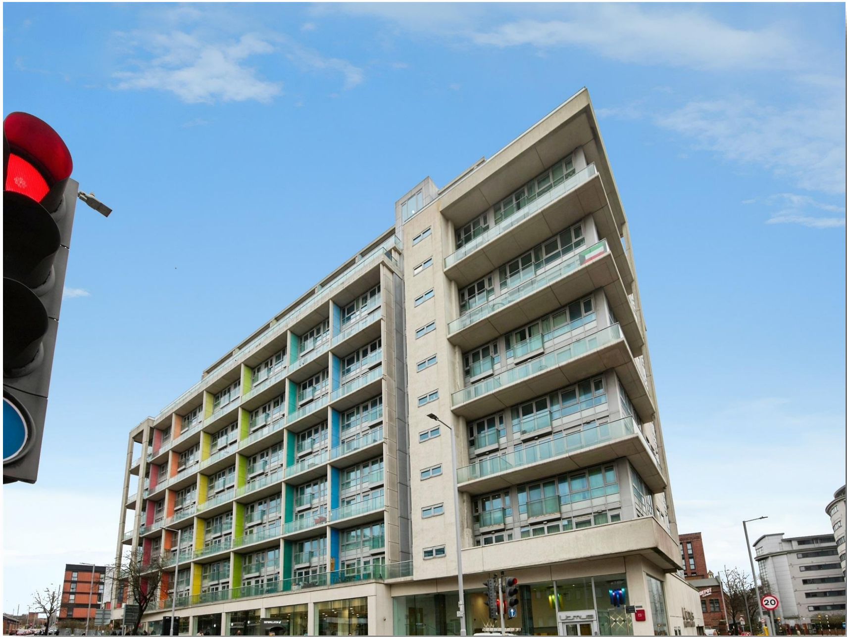
The Litmus Building Huntingdon Street, Nottingham NG1 3NX
